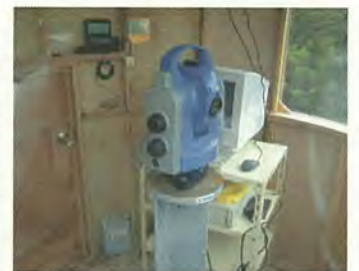
"Total Station" for automatic collimation
