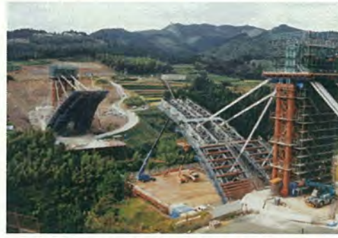
fig.1 Erection of Suspension supports
