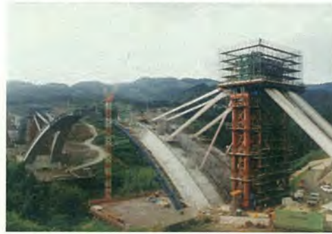
fig.3 Erection of Melan arches
