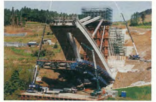
fig.2 Dismantling of Suspension supports
